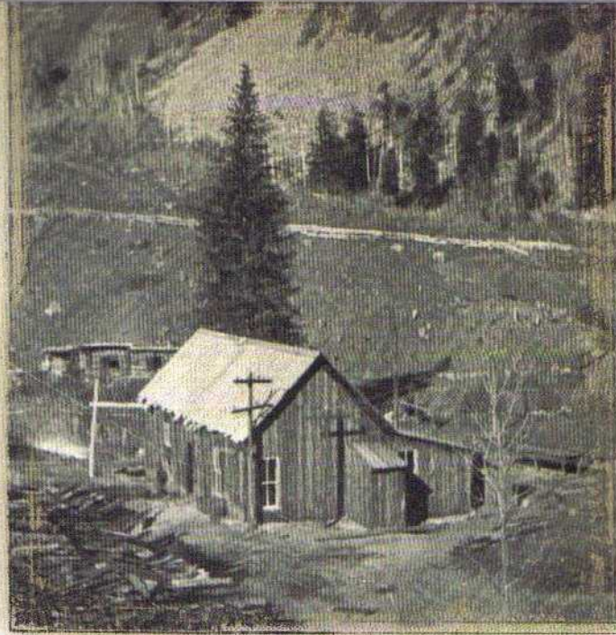
Aerial view of Western Colorado Power Co. Station at Ames, Colo. Photo Courtesy of Telluride Historical Museum, all rights reserved.
